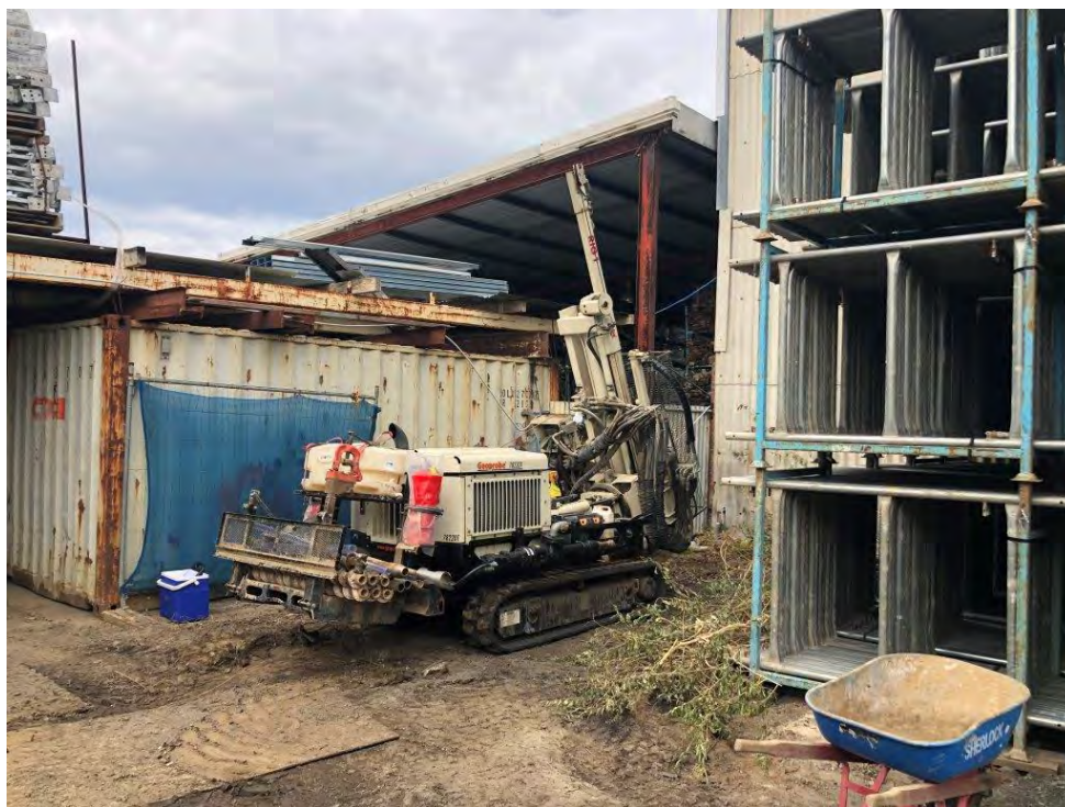
Photo 1: Drilling BH15/GW04 near former UST
