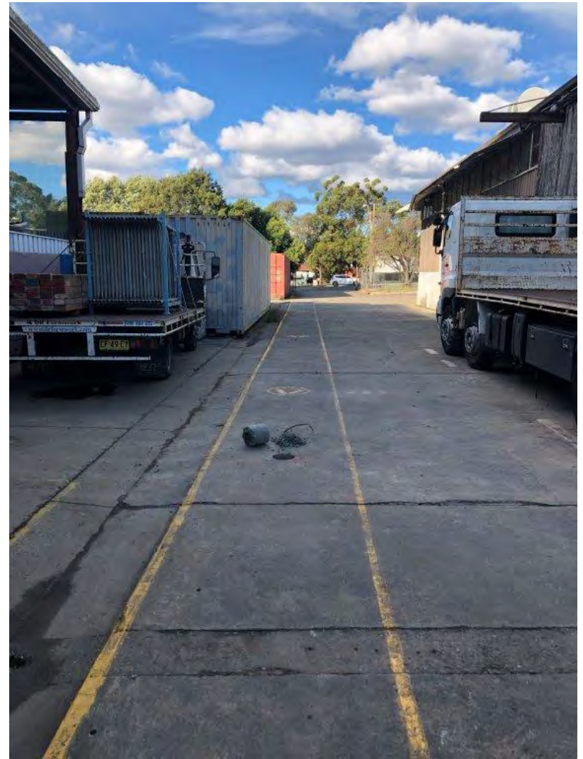
Photo 6: Assumed former settling pits area of Building #2. BH26 located over major stormwater or sewer pipe. Unknown layout of pipe network.
