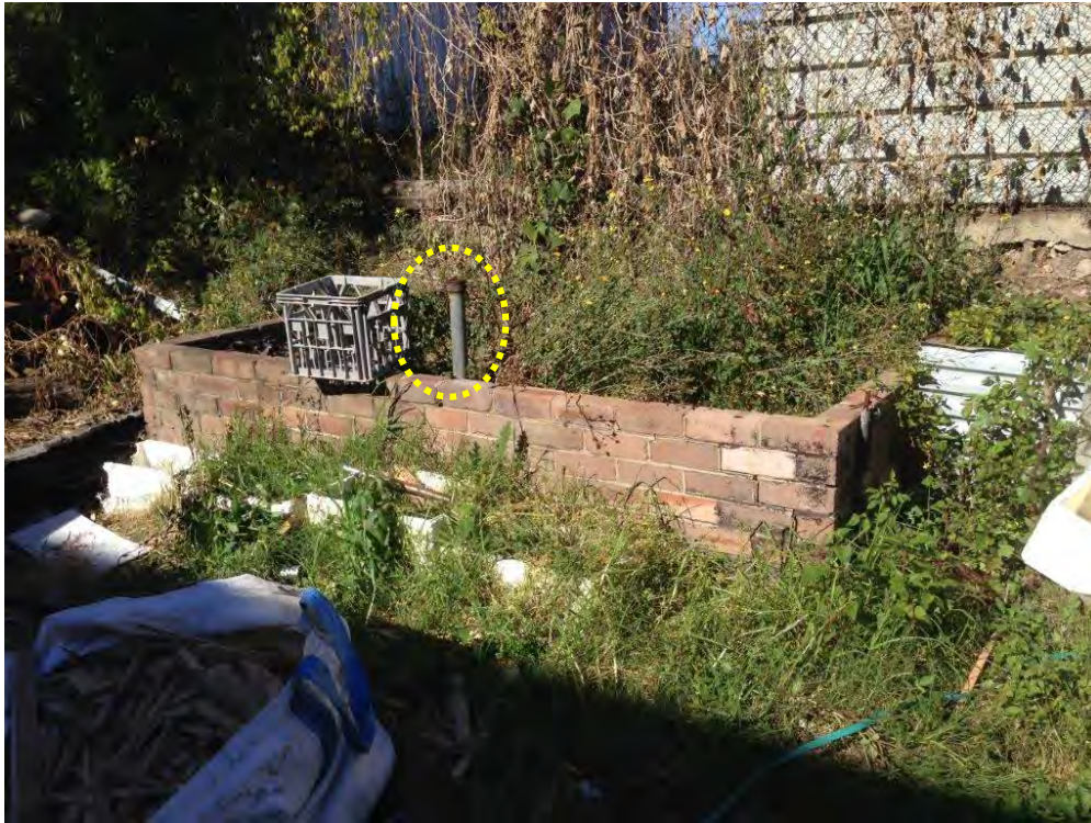
Photo 3: Former AST and bund (image from 2017). Unknown pipe visible.
